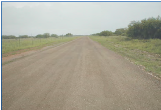
R3 roadbase applied on Delmita Road in Starr County, Texas.
